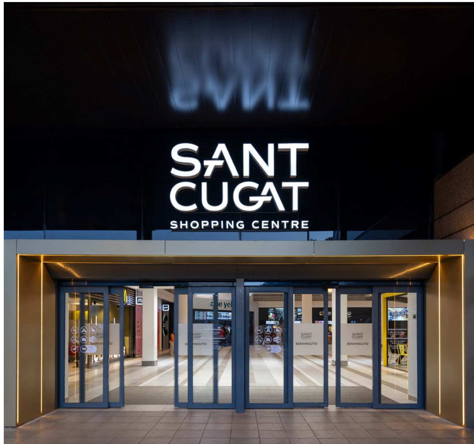
Sant Cugat Shopping Mall Location: Barcelona, Spain Project Management: DIR Project Architecture: MyG Architecture Lighting Design: Gisela Steiger Photo: Arnau Rovira
